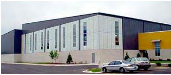
Preferred: dynamic roofline through changes in vertical plane, building element, colour and material
