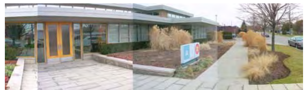
Building set close to the street with significant built frontage and articulated facade
