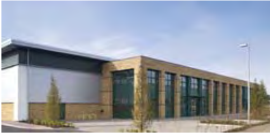
This building provides a purposeful change in material between the office and warehouse components
