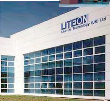
These signs are well integrated with the building
