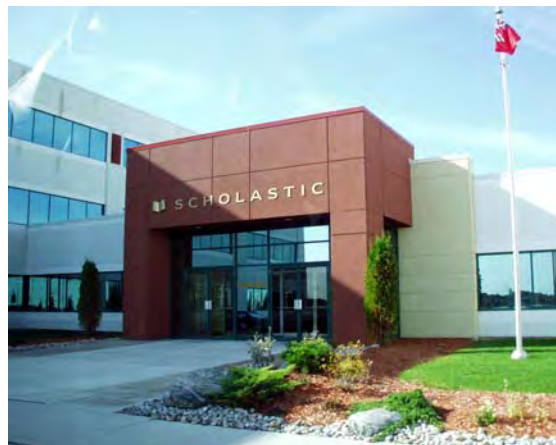
This building has a well defined entrance articulated by changes in plane, material and colour
