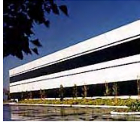
To be avoided: monotonous roof line
