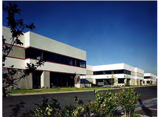
To be avoided: monotonous treatment of multiple building site
