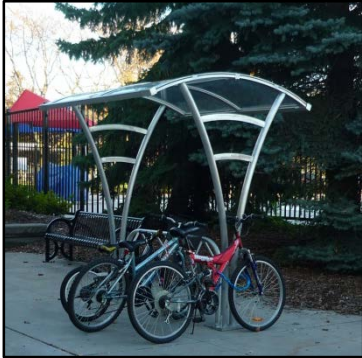
Figure 3 - Covered bicycle parking at Town Hall
