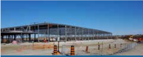
Amazon Fulfillment Centre - Structure
