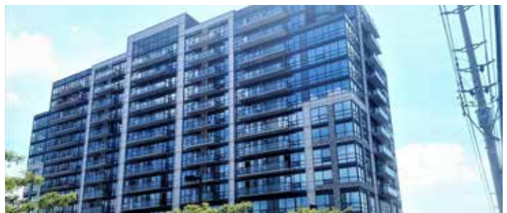
Exterior view of Parkland Ajax
