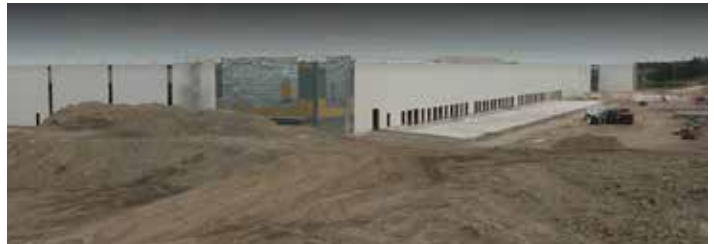
H&M Building Exterior
