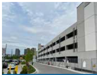
New Hospital Parking Garage
